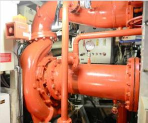
Built by Grandweld in 2009, Bourbon Agathe arrived at Grandweld facility for a modification job. The modification job involved design, installation and commissioning of external FiFi system according to BV class requirements for FiFi-1 notation.
